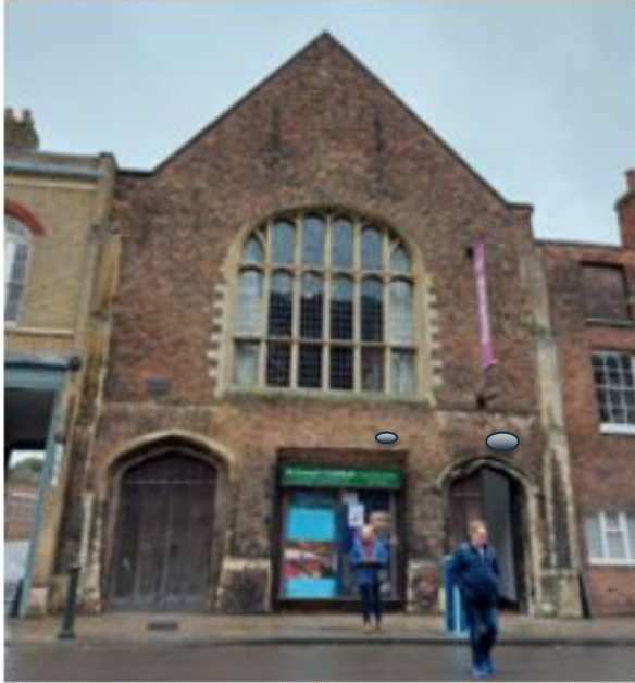
Existing Guildhall facade to King Street
